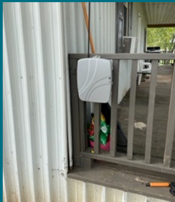
The contractor placed the Network Interface Device on the deck's rail. A union tech had to return to the customer and place it on the house where it belongs.
